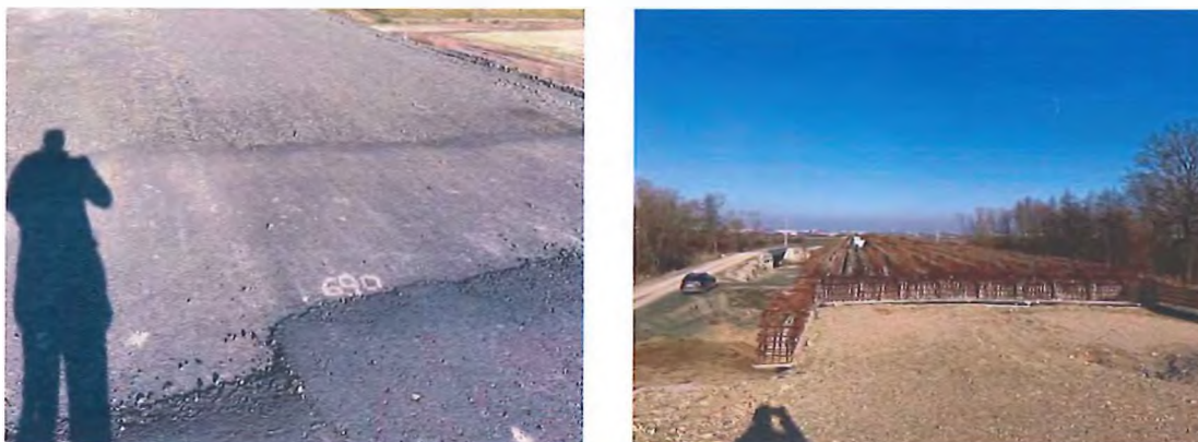
Fig. 6.5.33-3 Pod peste Bega: rampa sud
